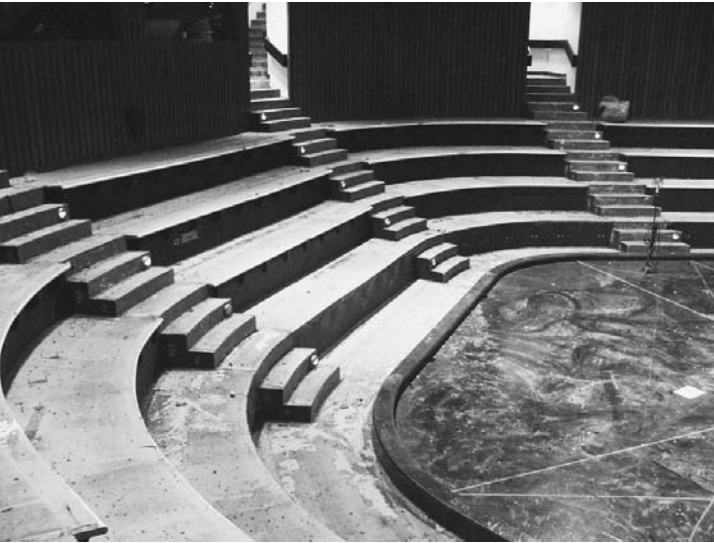
The Drama Theater, shown left before this summer’s renovations, was given a complete overhaul. The first steps were to scrape the ceiling and refurbish the walls. Right: By June 8, the old seats and carpet were removed from the theater. Sections of the concrete bleachers were dug out to create A.D.A. compliant platforms at house left and right.
